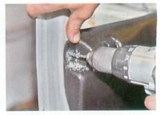
Trims are held by supplied fixing screws. Dave drilled 4 mm pilot holes into the door frame and 5 mm clearance holes in the GRP to take the screws.
