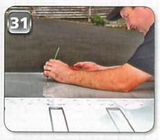
PICTURE 32 After carefully measuring and drilling a pilot hole, a tank cutter was used to drill a larger hole in the ribbed beneath so that the fixing nut could be fitted - and the shark's fin aerial swam into view.
